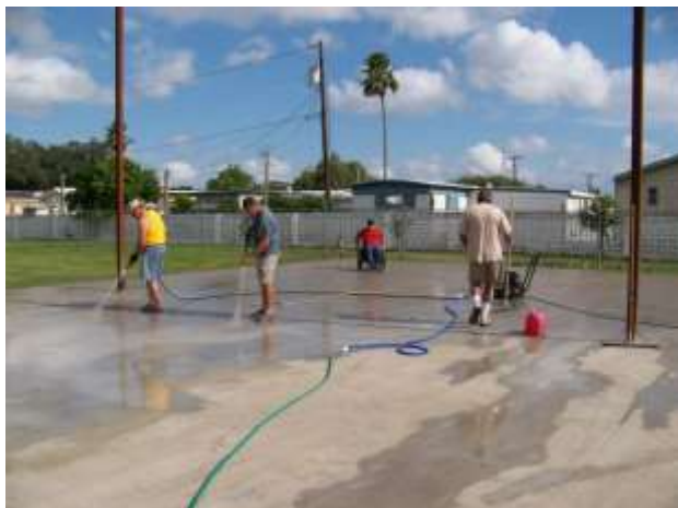
Workers power wash surface clean after treating concrete
