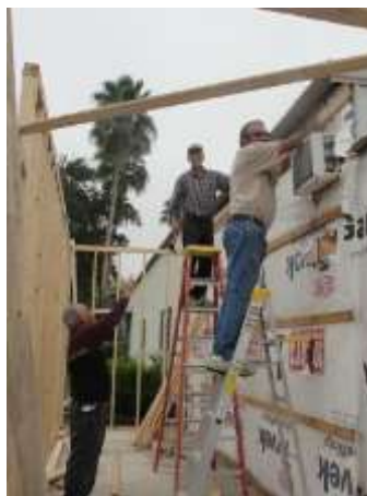
Additional woodshop space takes shape as walls and ceiling are built
